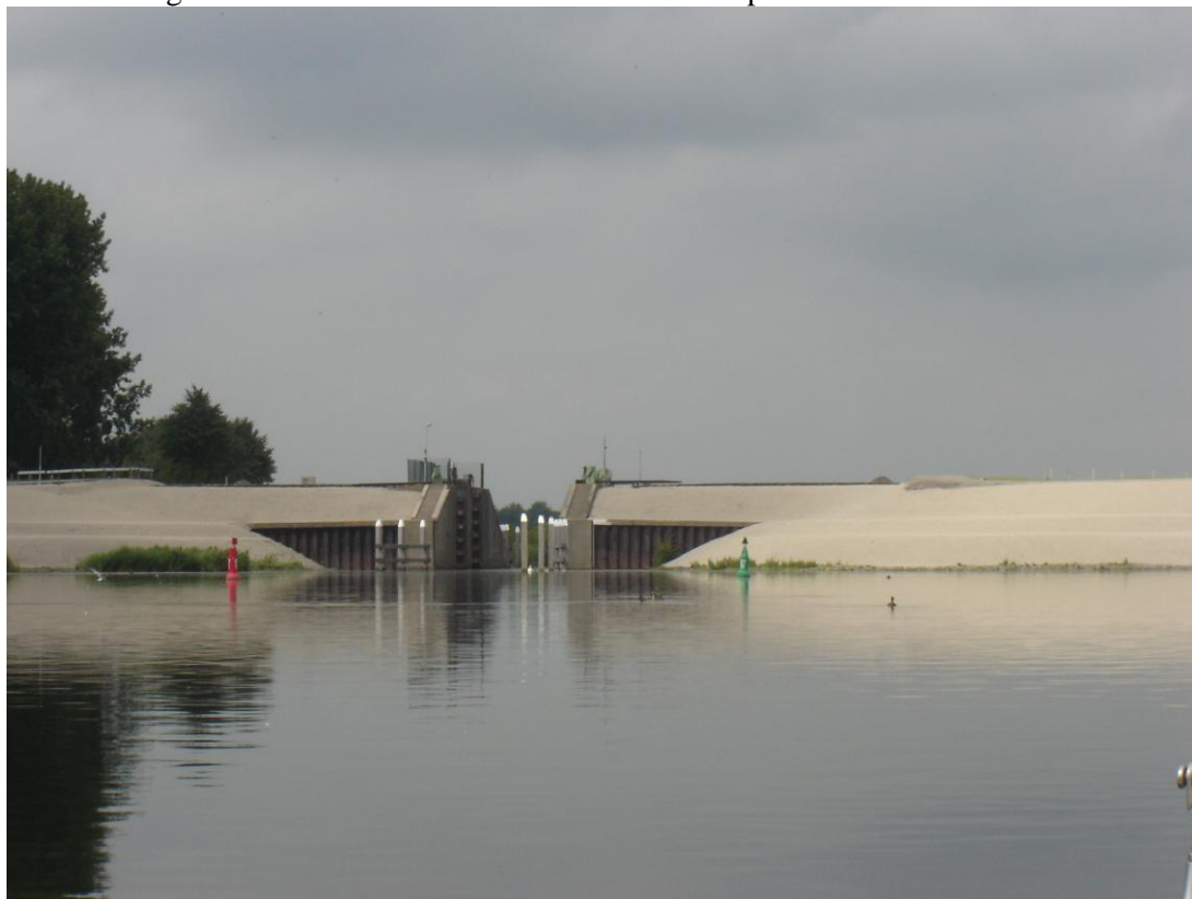
Photo 1. Sluice of Oude Tonge
