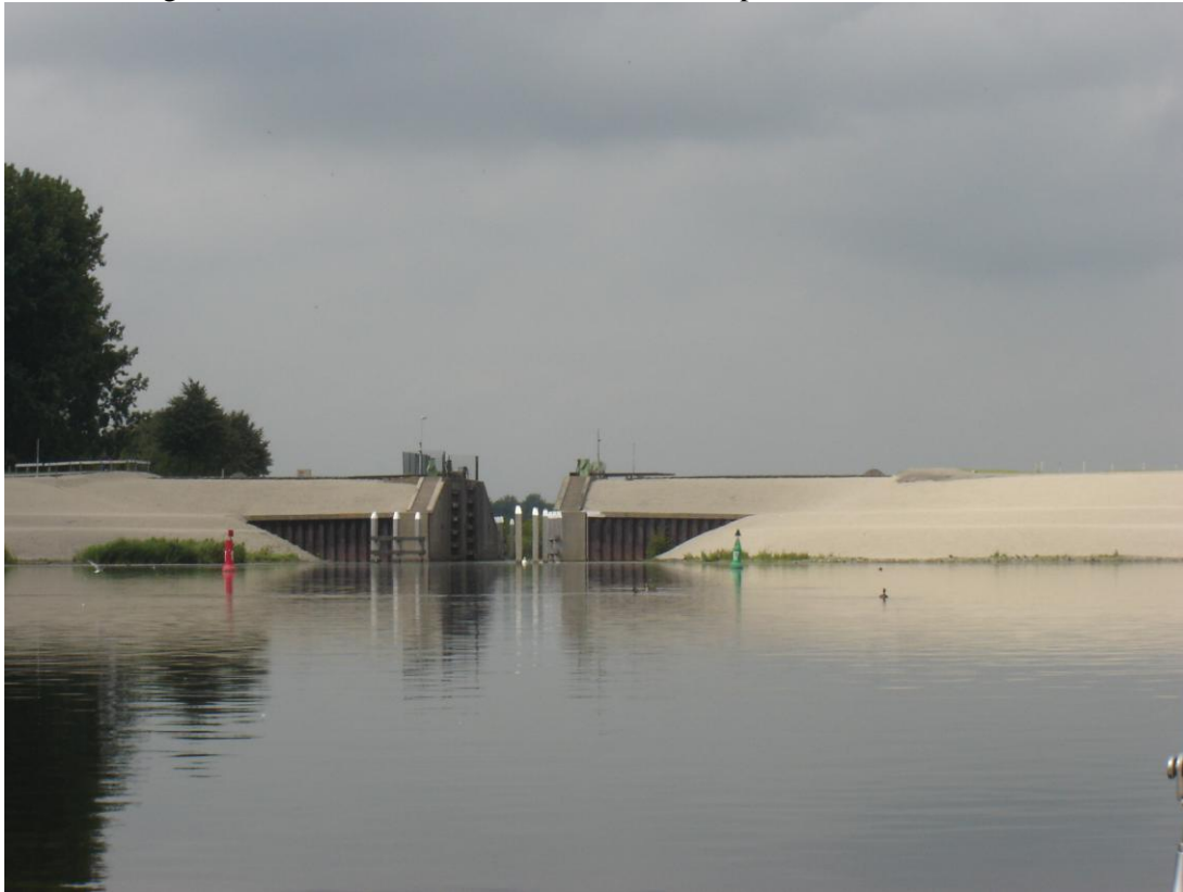
Photo 1. Sluice of Oude Tonge
