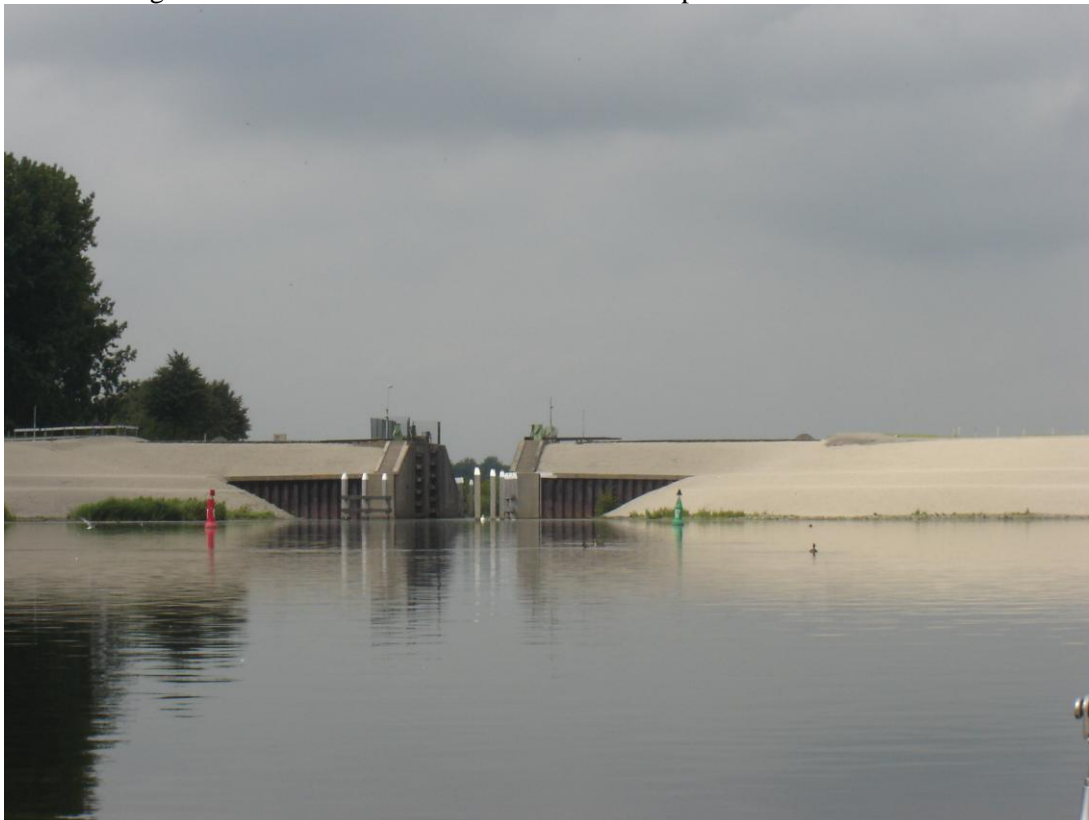
Photo 1. Sluice of Oude Tonge
