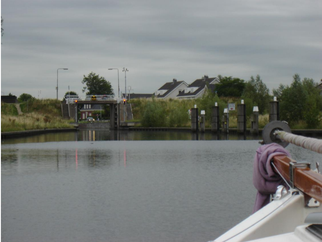
Photo 7. 19 th century lock, the entrance of the river Linge and Merwede-canal at Arkel.
